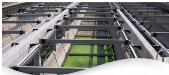
Sludge and Oil Remove system SCRAPER (Scrapers System)
