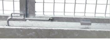
Locking mechanism at the bottom of the doors
