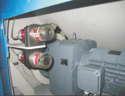
Automatic central lubrication with adjustable interval
