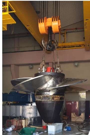
turbine assembly HPP ĐALE, Croatia
