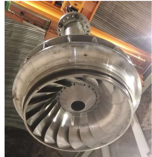
turbine disassembly HPP DUBROVNIK, Croatia
