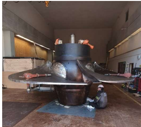
turbine disassembly HPP SPJUTMO, Sweden
