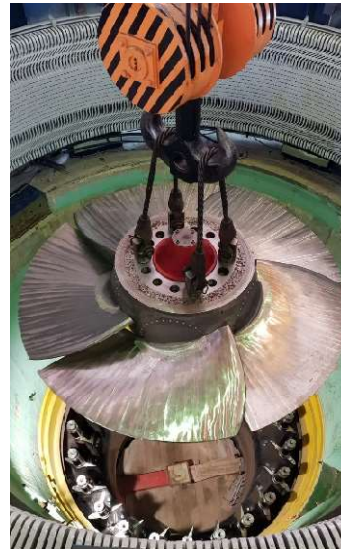
turbine assembly HPP ĐALE, Croatia
